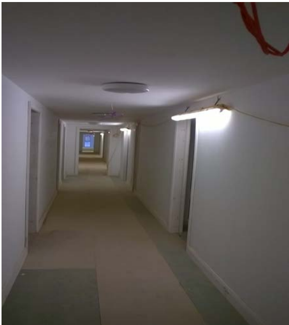
Internal corridors to Block C/E
