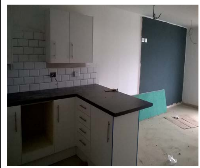
Kitchen fit out to Block E
