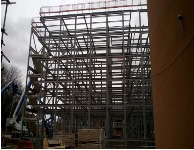
Completion of last staircase and steel frame to Block D
