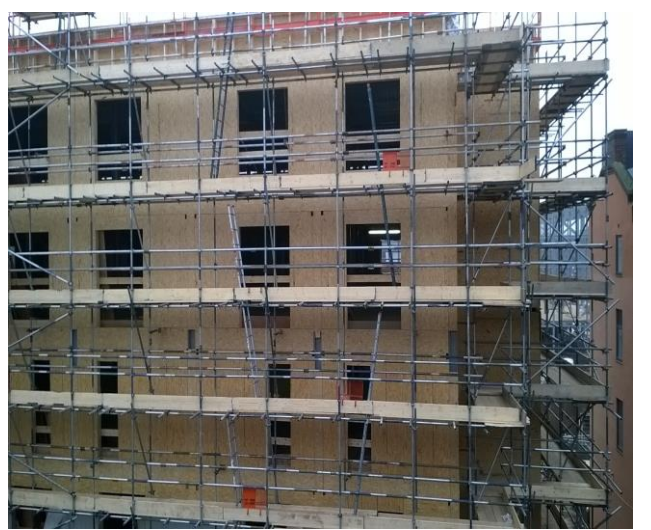
External envelope to Block B
