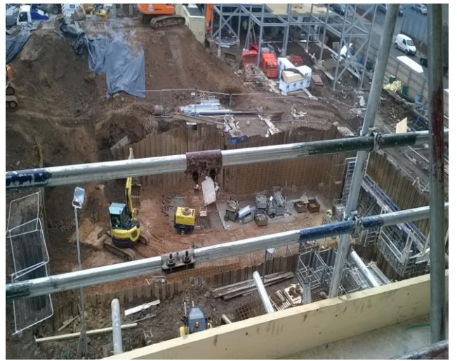
Second basement works to Block D
