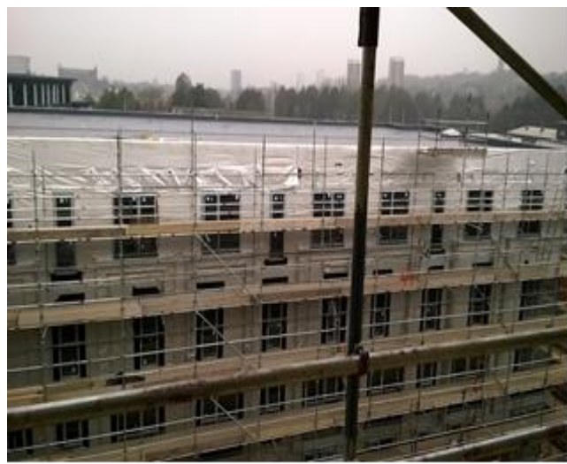
External envelope to Block C
