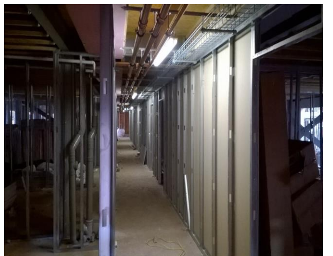
Internal corridor to Block B
