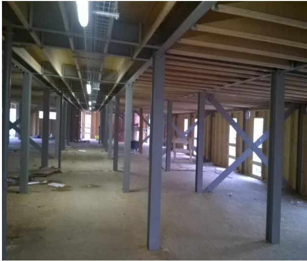
Top floor of Block B
