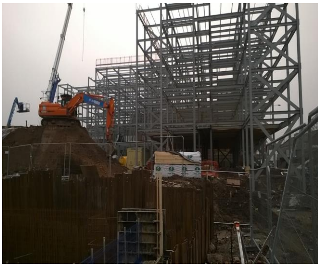
Steel frame to Block D
