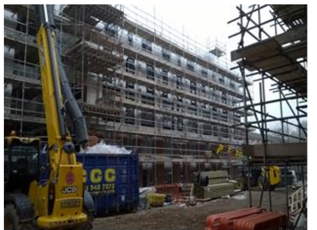
External envelope to Block C
