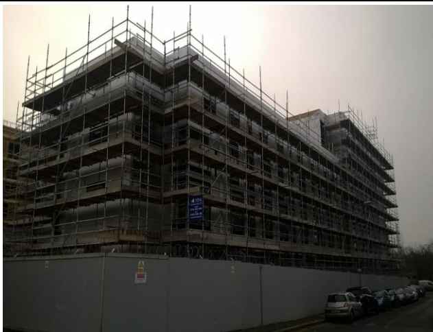
External envelope to Block C and E
