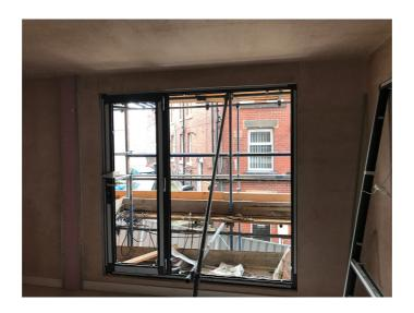
H. Typical 1<sup>st</sup> Floor/Second Floor Progression. Windows installed and 'Mist-coat' completed.
