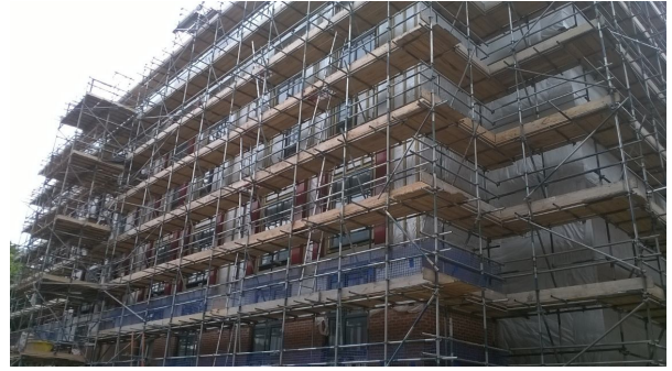
External façade to Block B
