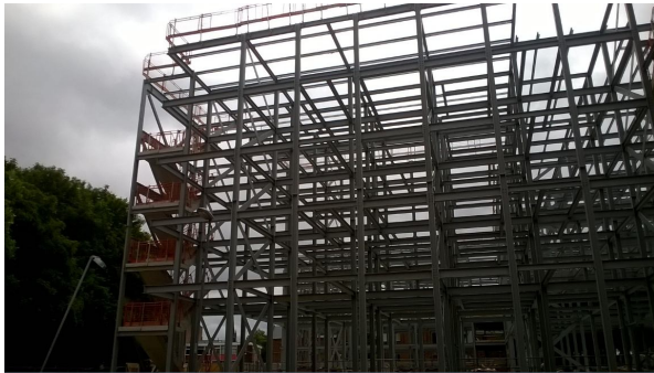
Completion of frame and staircases to Block D
