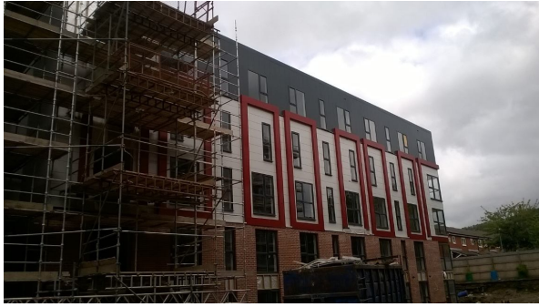
External façade to Block C with Scaffold now removed
